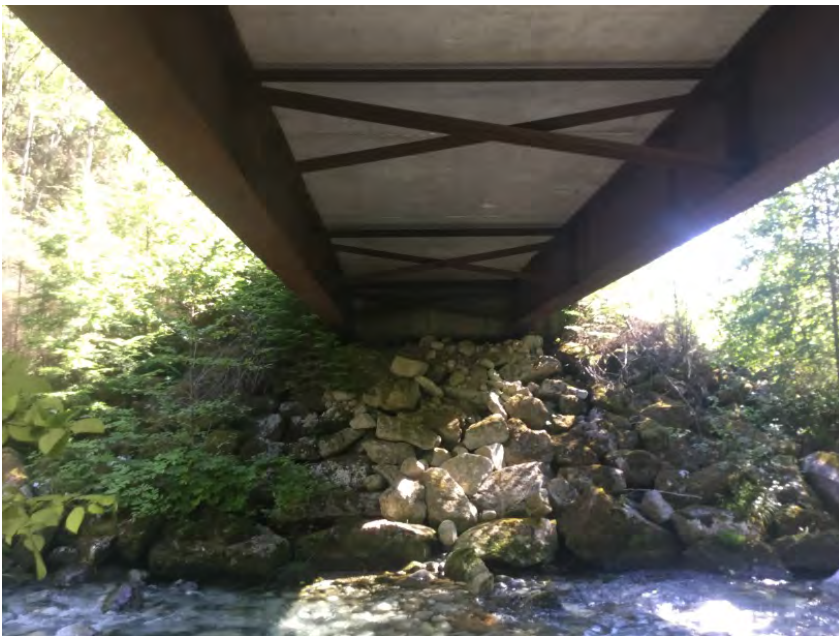
Left Bank Abutment
