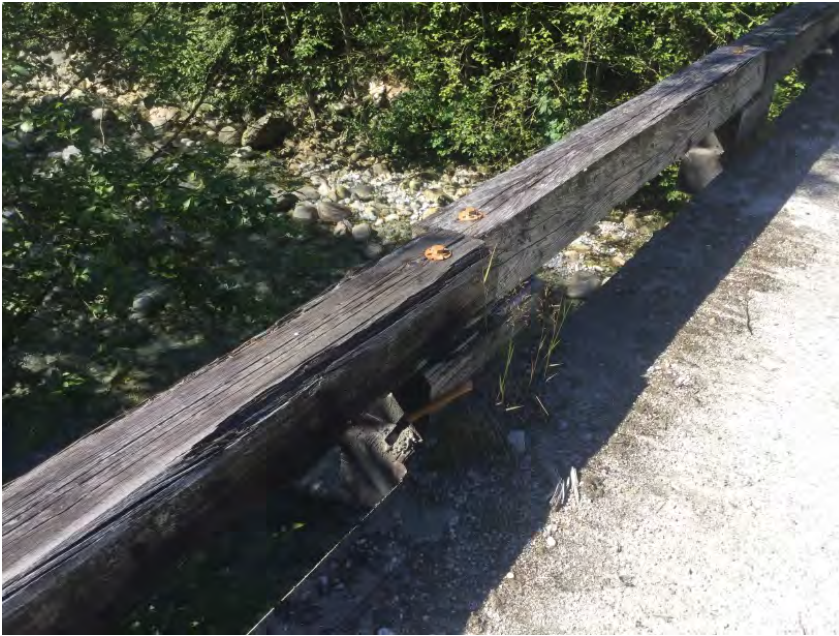
Deteriorated Guardrail
