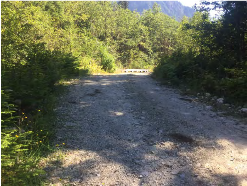
Right Approach Facing Bridge
