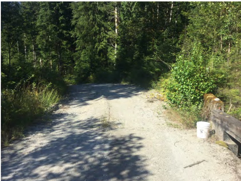
Right Approach Facing Away From Bridge
