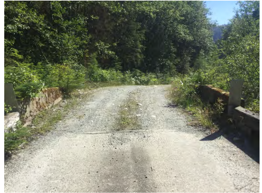
Left Approach Facing Away From Bridge
