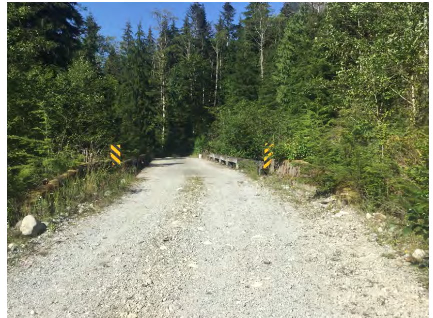
Left Approach Facing Bridge
